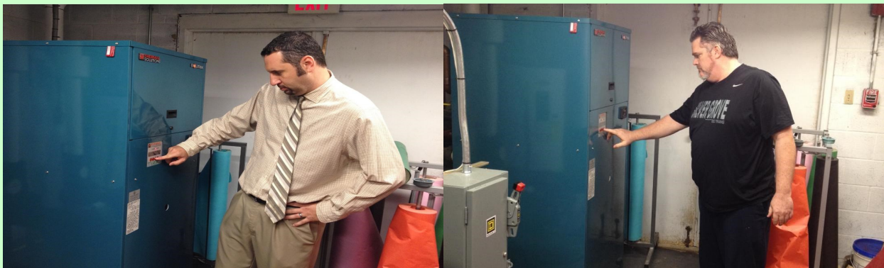
When the boiler is needed Principal Wes Murray and Custodian Pat Gossett work as a team. Wes will turn the system on in the morning and Pat will set it back during unoccupied times.
